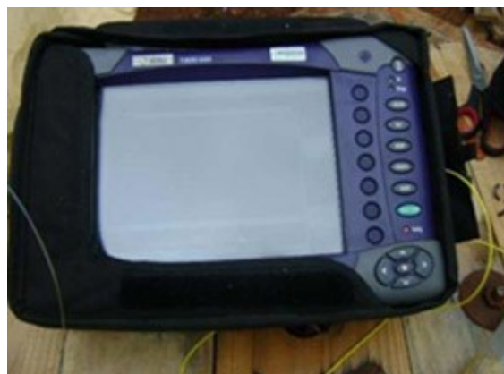
On site fiber testing
