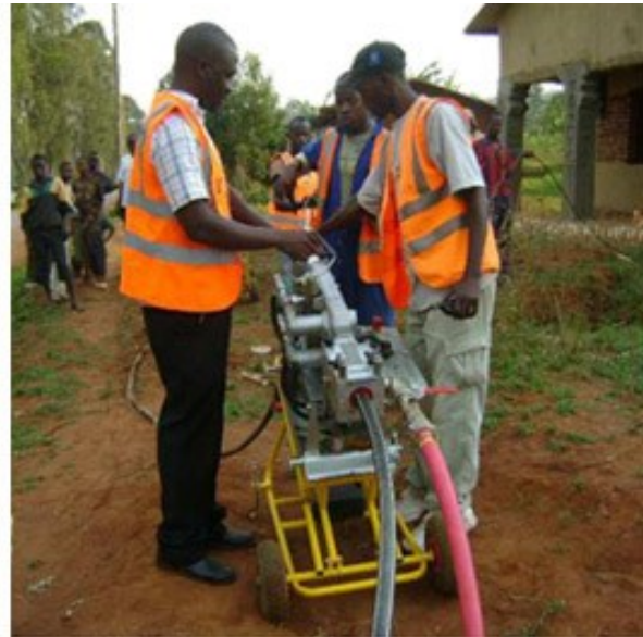
Fiber blowing process
